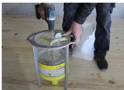
Put the chippings into the CLT BOX – CEILING FS using a cordless screwdriver
