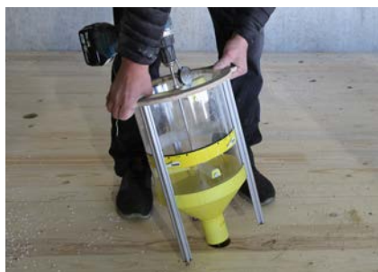
Place the EASY FILL filling aid over the opening of the CLT BOX – CEILING FS
