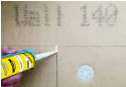
Closing the installation joints by means of FDM WALL.
