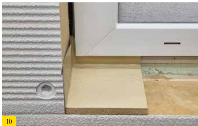
The 5 mm projection of the lip must form a U between the edge of the window and the wood fiber board.
