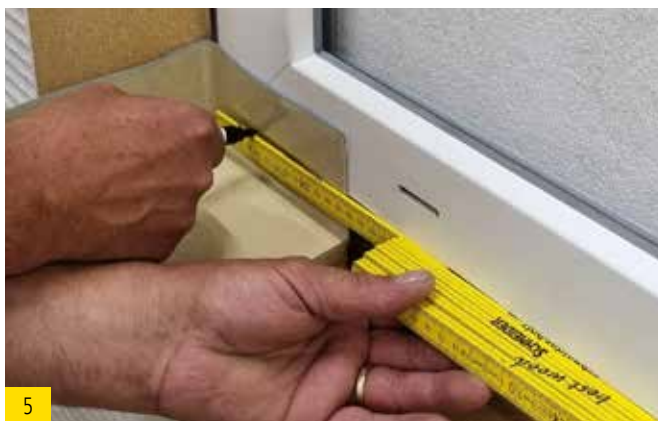
5 Mark the height of the lip of the sealing corners at the lower edge of the window.
