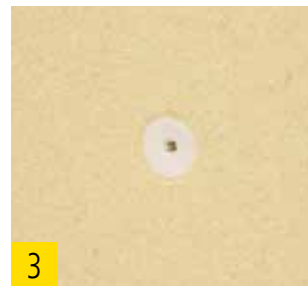
3 Flush-mounting of the spiral anchor.
