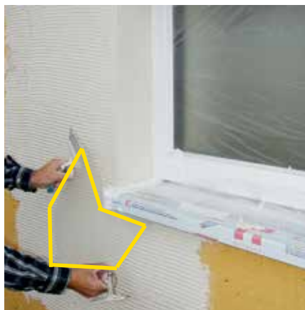
Embedding of reinforcing arrow.
