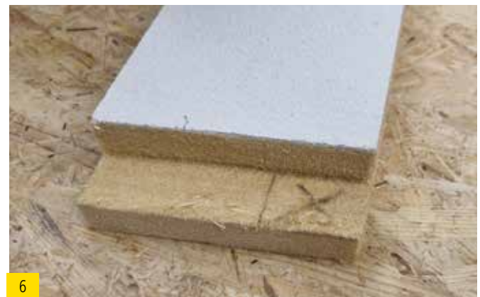
Saw out the marked area.
