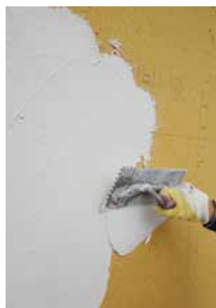
Application of adhesive and reinforcing mortar (UP).
