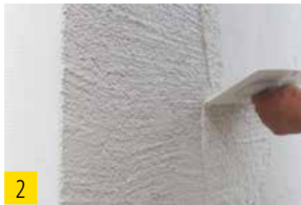
The final render is applied by means of a trowel and then skimmed to grain size.
