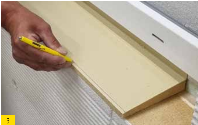
3 Mark sealing wedge with appropriate depth.
