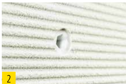
2 The screw-in plate has to be inserted by about the thickness of the plaster layer.
