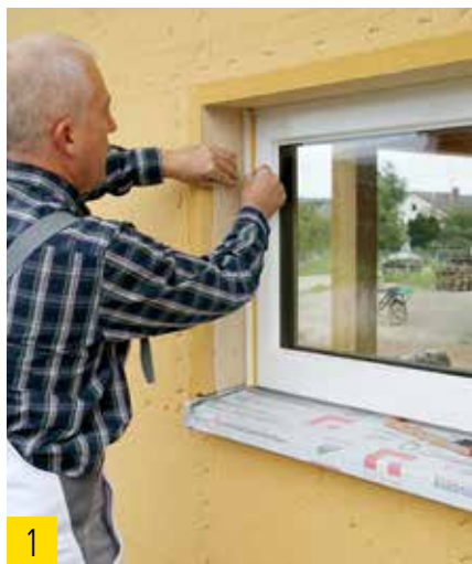
Affix telescopic plastering strip.
