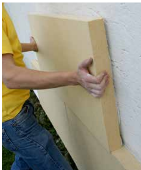
Application of WALL 140 by means of a light sliding movement.
