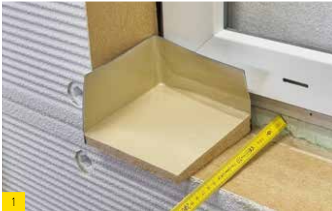
1 Measure depth of window sill.
