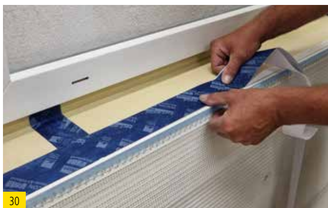
Affix the best wood window sill render stop bead to the sealing level with TESCON VANA.
