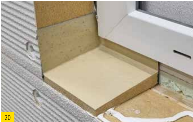
Important: Make sure that a "U" is formed again between the window frame and the wood fiber board (see picture no. 10)
