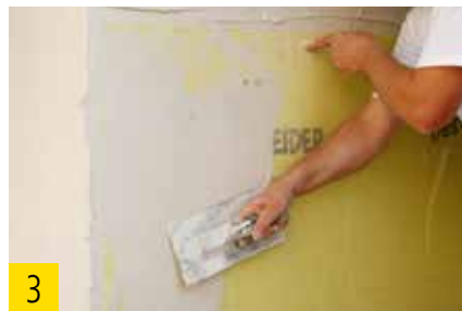
3 Wet embedding of the best wood reinforcement fabric.
