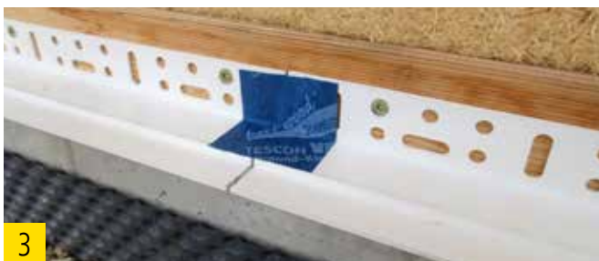
3 Bonding of the joint by means of a fabric tape.
