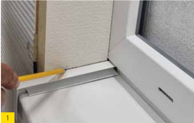
Notching of the 40 mm reveal board.
