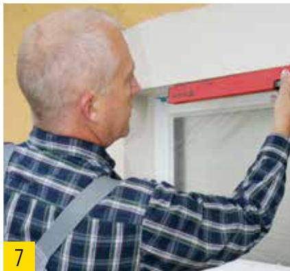
Horizontal and vertical alignment of the corner bead with fiber mesh.
