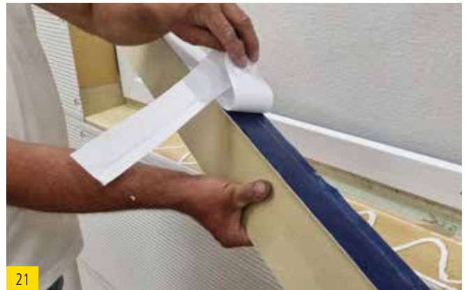
Pull off the adhesive tape from the sealing wedge which was cut to size previously
