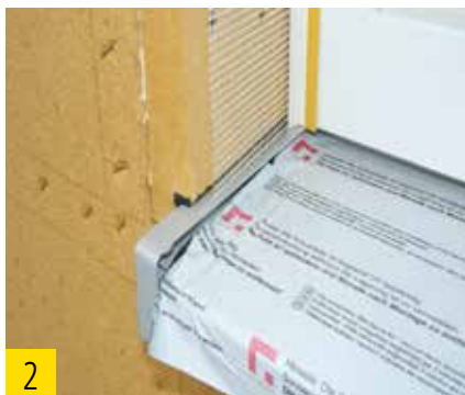
Architrave bead with telescope function sits flush to the inner edge of the window sill end piece.
