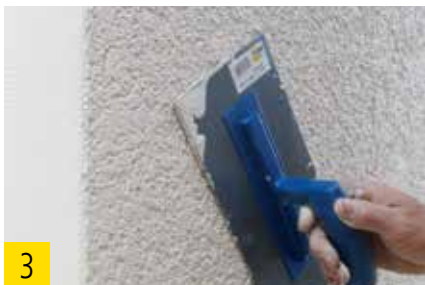
Structuring of the final render by means of a trowel.
