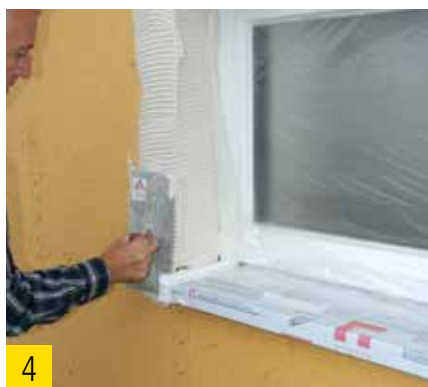
Application of adhesive and reinforcing mortar (UP) to the window reveal and the outer edge.
