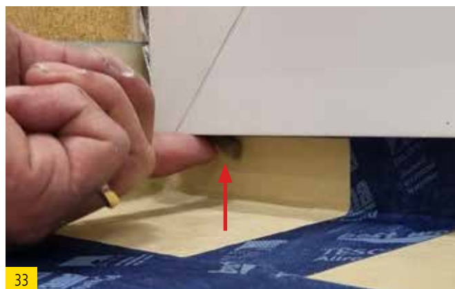
Affix the sealing cord in the corners beneath the window frame in the cavity so that it is closed.
