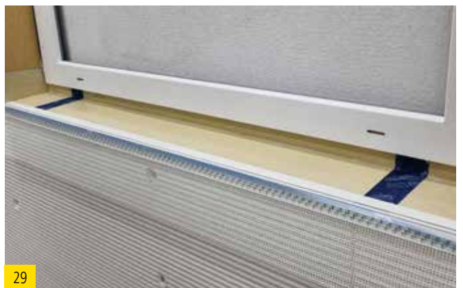
Fit the best wood render stop bead between the reveals in a central position.
