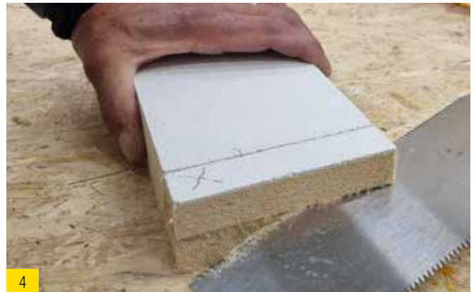
Scribe 20 mm and mark what is to be cut out.
