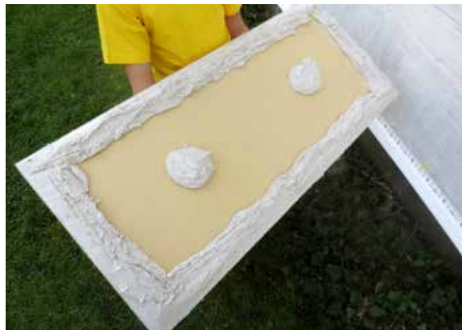
Application by means of the spot-and-bead method.
