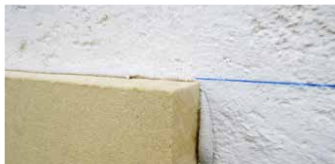
Horizontal alignment of WALL 140 boards by means of a marking chord.
