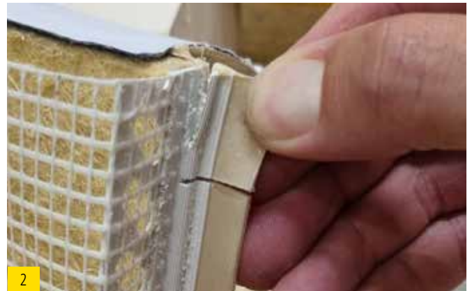
Shorten render stop bead including mesh web to marked length.
