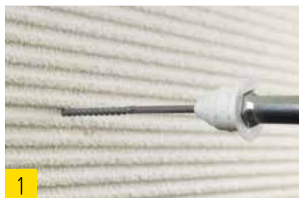
1 Install screw-in anchor for insulation boards H35 (in the approval procedure) with the best wood mounting tool.
