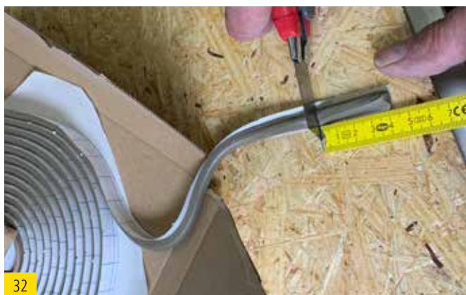
Cut off 4 cm of the sealing cord.
