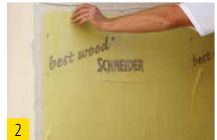
2 Application of best wood reinforcement fabric.
