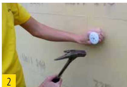
Application of the screw-in anchor.
