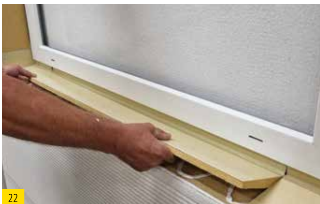
Push in the sealing wedge between the corners, fitting exactly
