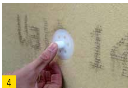
Application of the closing plug.
