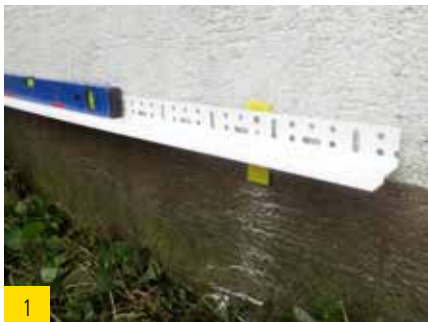
1 Base rail must be aligned and fastened horizontally.
