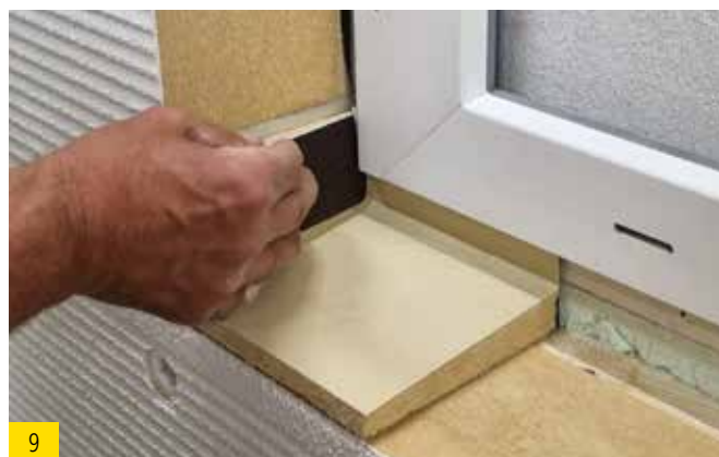
Insert both corner pieces and neatly press into the corner of the window sill using a tool (such as a wooden wedge).
