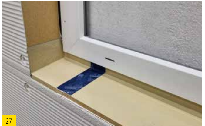
Firmly press down the TESCO VANA - use the same procedure at both joints.
