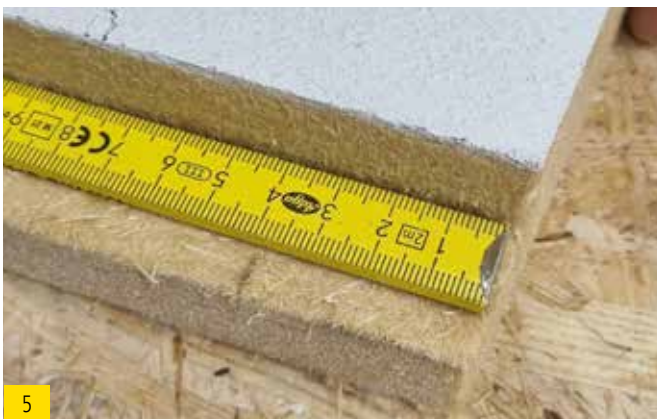
Measure 40 mm for notching the rear corner at the window.
