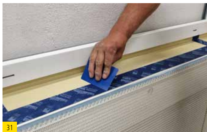
Smoothen the adhesive tape with a squeegee.
