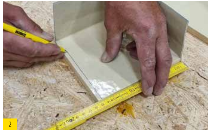
2 Mark sealing corner with appropriate depth.
