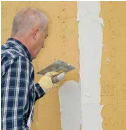
Application of adhesive and reinforcing mortar (UP).
