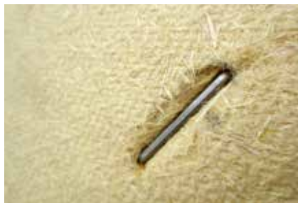
Stainless steel broad back staples have to be countersunk approx. 1 mm into the best wood WALL 180.
