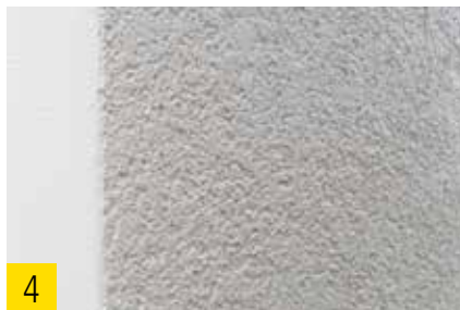
Ready structured plaster surface.
