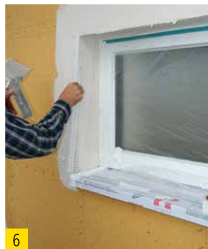
Application of corner bead with fiber mesh.
