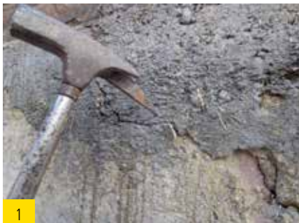
1 Remove all loose plaster.
