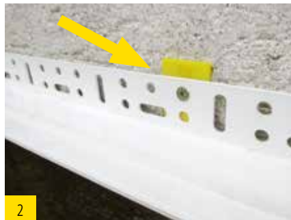
2 Distance adjustment at the base rail.
