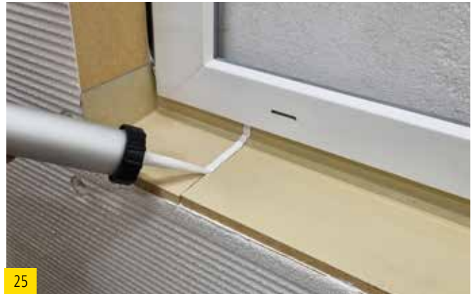
Seal the joint between the sealing corners and the sealing wedge with best wood FDM WALL.
