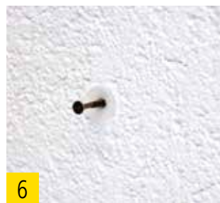
6 Fastening of the attachment piece by means of a 4–5 mm screw.
