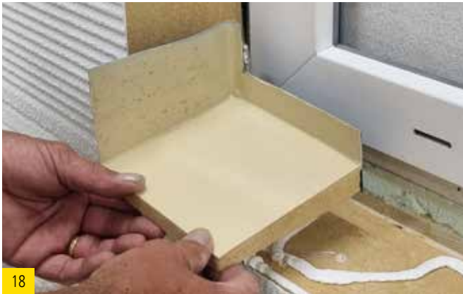
Position the sealing corners in both corners.
