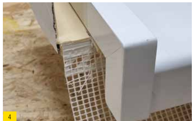
Render stop bead and window sill with same length.
