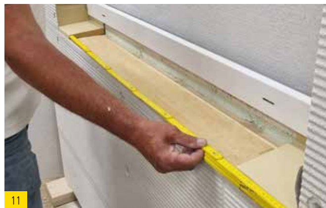
Measure the gap between the left and right sealing corners and shorten the sealing wedge (middle section) to the correct length.
