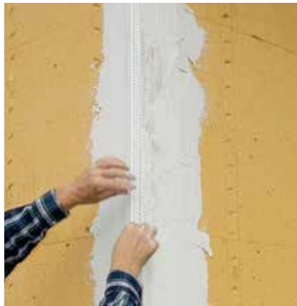
Application of corner bead with fiber mesh.
