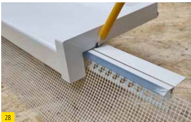
Shorten the best wood window sill render stop bead to the length of the window sill, including the end pieces.
