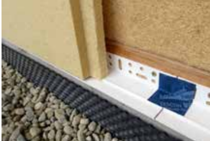
Cut off the groove side.
