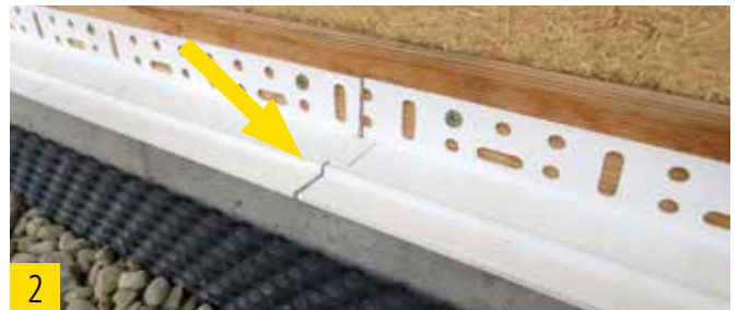
2 Installation of butt joint connectors at all longitudinal ends.
