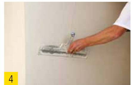
4 Embedding of the best wood reinforcement fabric.
