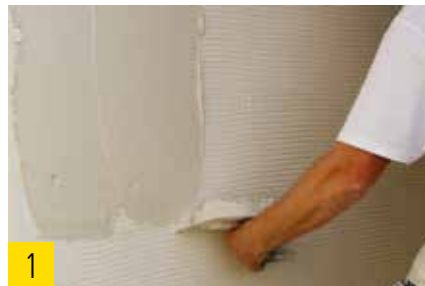
1 Application of vertical coating.
