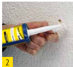
2 Application of best wood FDM WALL under the anchor plate.
