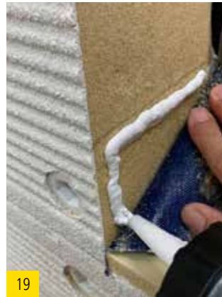
Apply best wood FDM WALL to the front. With the aid of a wedge, then press the sealing corner all the way in between the edge of the window and the wood fiber board.
