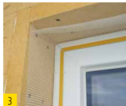
Architrave bead mitered in the edge.
