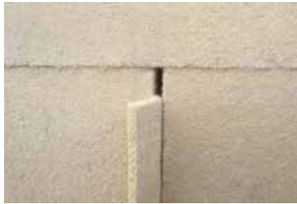
Closing the installation joints by means of strips from WALL 140/180.
