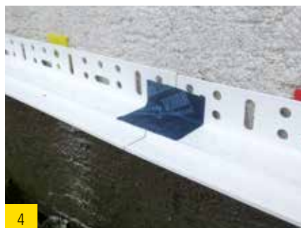
4 Bonding of the joint by means of a fabric tape.
