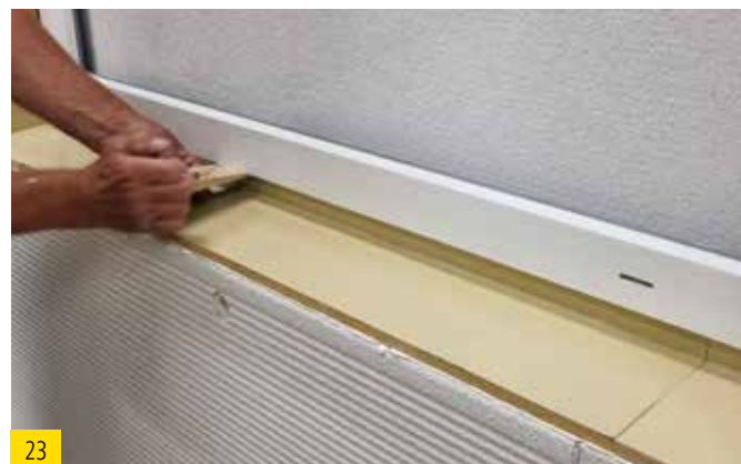
Also firmly press on the adhesive strip below the window frame using a tool (such as a wooden wedge)
