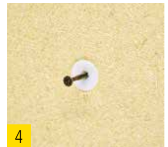
4 Fastening of the attachment piece by means of a 4–5mm screw.
