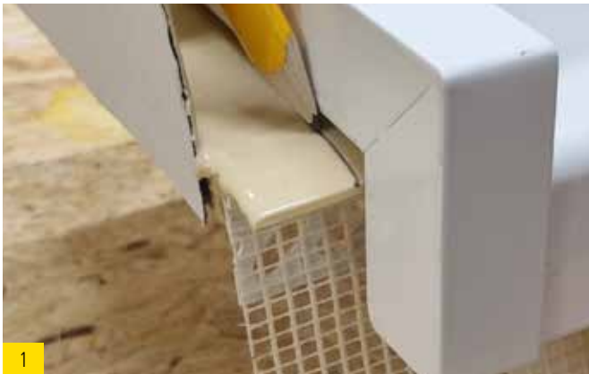
Mark window sill length on left and right sealing wedge.
