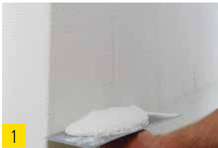
The final render is applied by means of a trowel and then skimmed to grain size.
