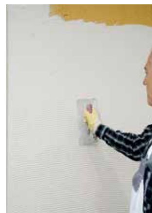
Application of serrated layer of mortar.
