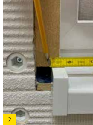
Scribe 20 mm and mark what is to be cut out.
