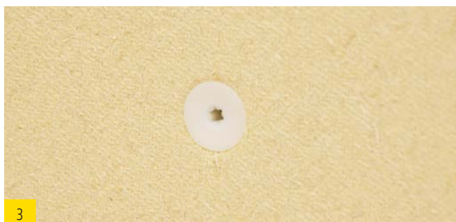
3 Flush-mounting of the spiral anchor.
