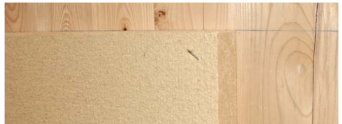
Horizontal alignment of the first row of panels by means of a marking chord.
