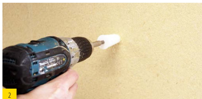
2 Insertion of the spiral anchor by means of a TORX T40 into the unrendered wood fiber insulation board.
