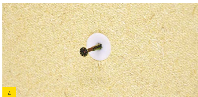
4 Fastening of the attachment piece by means of a 4–5 mm screw.
