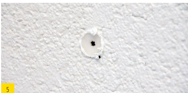
5 Remove any excess FDM WALL between plaster and spiral anchor.
