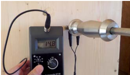
Wood moisture content \leq 18\% .
