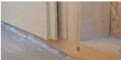
Cut off the groove side.
