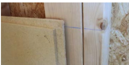
Horizontal alignment of the first row of panels by means of a marking chord.
