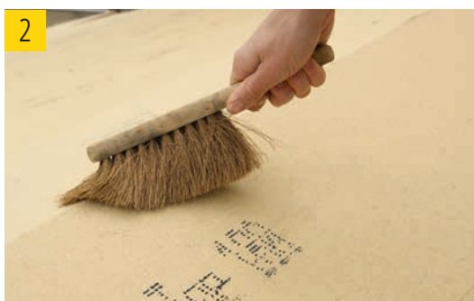
(2) The underlay must be dust-free to establish a permanent connection. Remove dust and sawdust from the underlay using a brush or compressed air.
