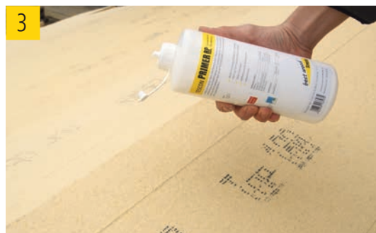
(3) Apply TESCO PRIMER RP in the width of adhesive tape with a brush (4) to the TOP or use the application tool TENAPP (5).
