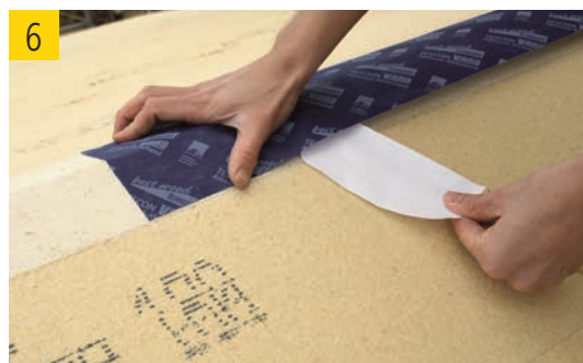
(6) Stick TESCO VANA adhesive tape onto the joint to the dry or wet primer and press down firmly.
