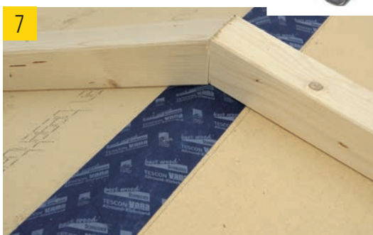
(7) The ridge joint is sealed and counter battens are secured to the wood fiber boards.
