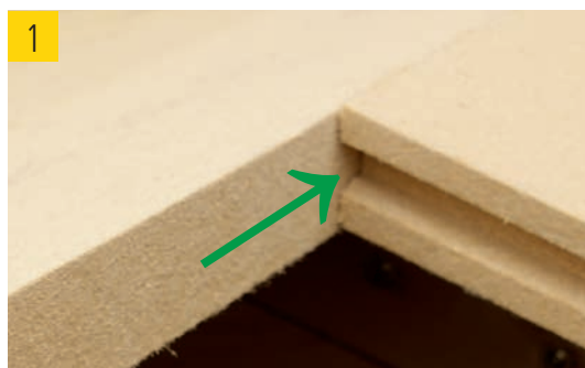
(1) best wood wood fiber insulation must be laid free of joints and mitered to prevent thermal bridges in the insulation.
